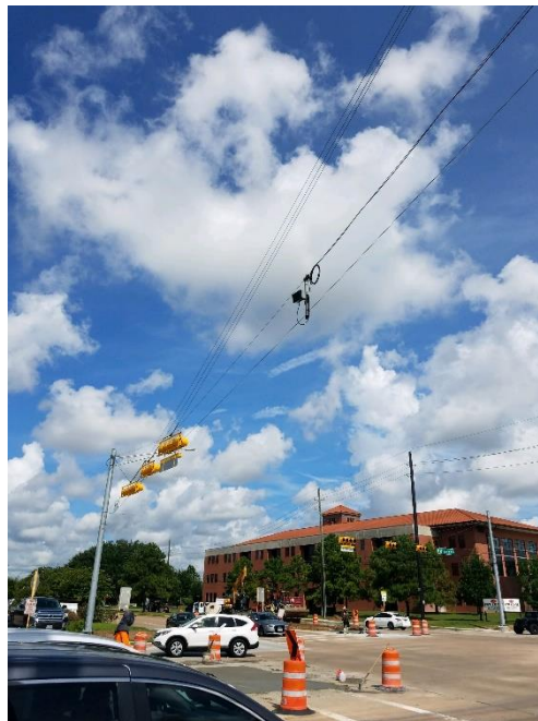
Figure 3-7: Dual Span wire installation
