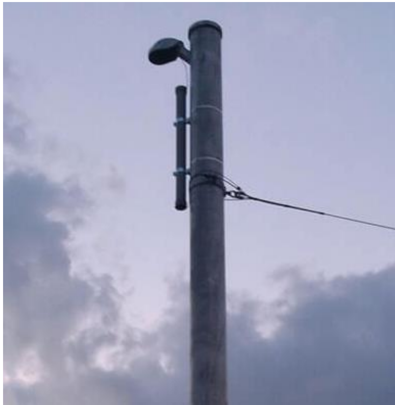
Figure 3-8: Strain Pole installation
