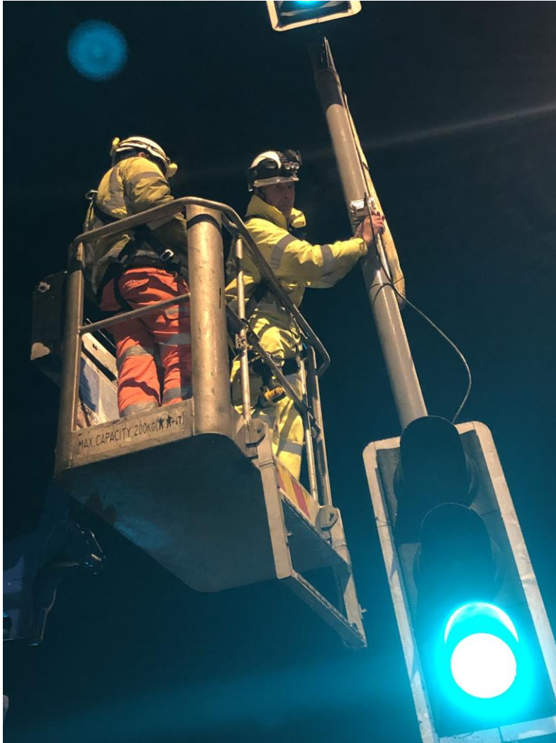
UMRR-11 Type 45 installed at 6m mounting height on Signal Pole 4
