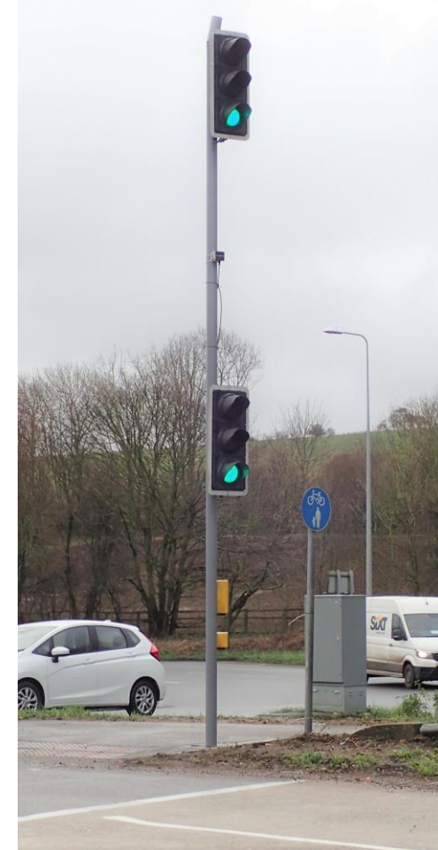
UMRR-11 Type 45 installed at 6m mounting height on Signal Pole 4
